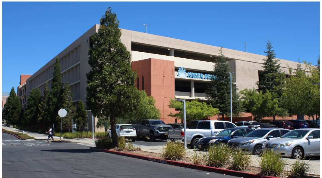
Kaiser Permanente Roseville Medical Center on Douglas Boulevard.
