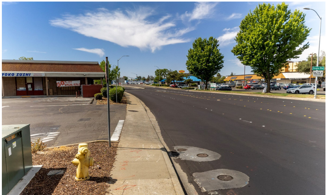
The four-foot sidewalks on Sunrise Avenue have no separation from the roadway and are bordered by large parking lots.
