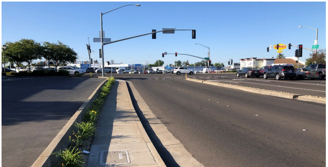
Sidewalks along the major commercial corridors in the Plan Area are generally 4 feet wide with no break between the sidewalk and the street.
