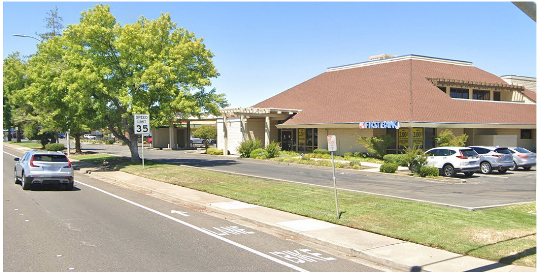
Existing Class II bike lanes on Douglas Boulevard.
