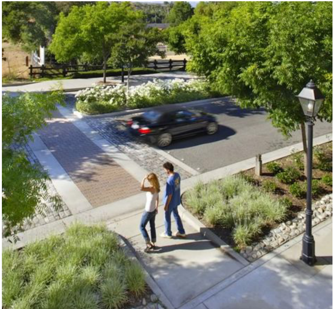
Color, material, and striping pattern variations applied to crosswalks reinforce the distinction between the pedestrian pathway and the road.
